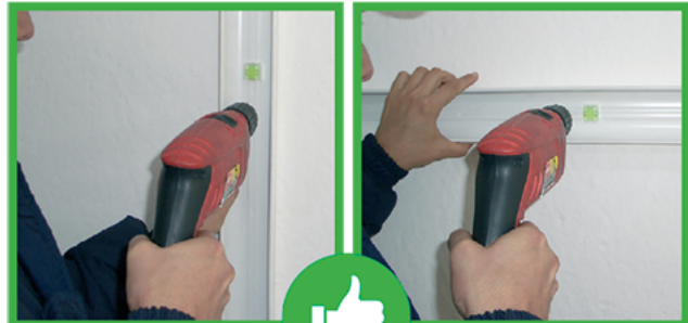
Duct installation with built-in level
