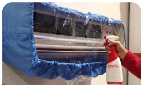
Battery cleaning with protective cover
