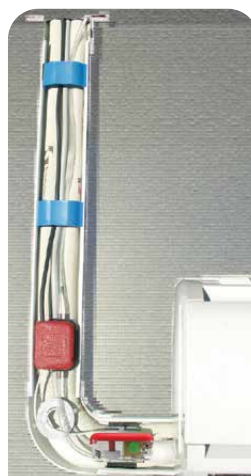
Laying pipes and pump
