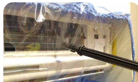
Battery cleaning through cleaning machine hole
