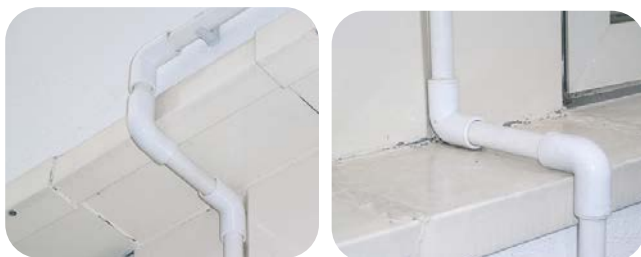
Example of installation with rigid TCR pipe and accessories
