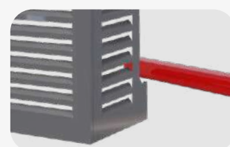
Preparation for passage conduit pipe and wiring
