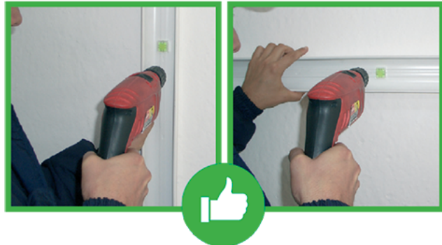
Duct installation with built-in level
