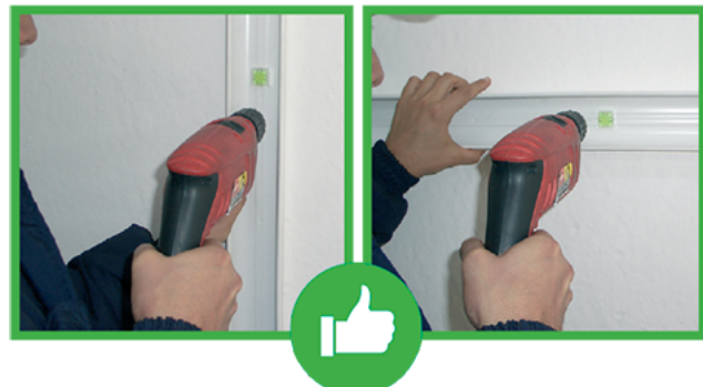
Duct installation with built-in level
