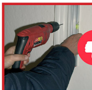
Duct installation without built-in level
