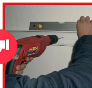
Duct installation without built-in level
